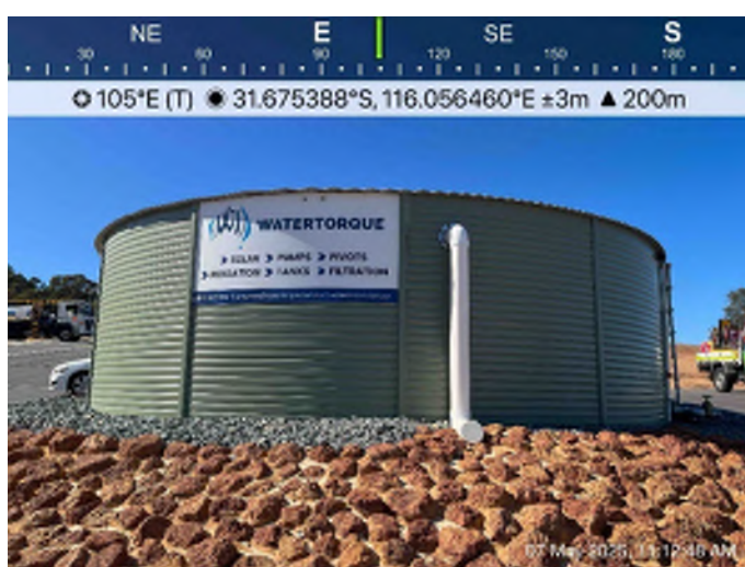
Plate 4: Compliant 100 kL fire water tank within Yarrimbah Drive road reserve (facing east)
