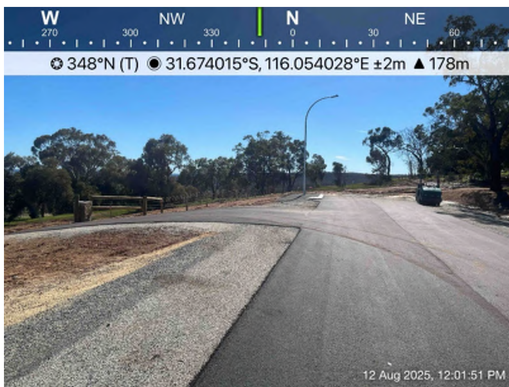
Plate 6: Compliant Grevillea Road cul-de-sac and hammerhead turnaround
